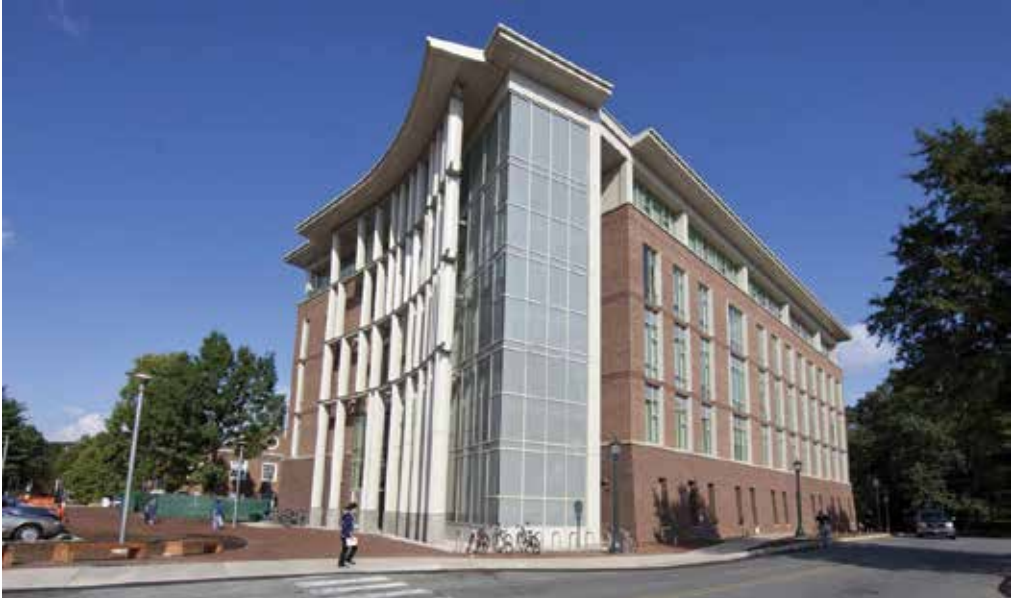
Rice Hall Information Technology Engineering Building
